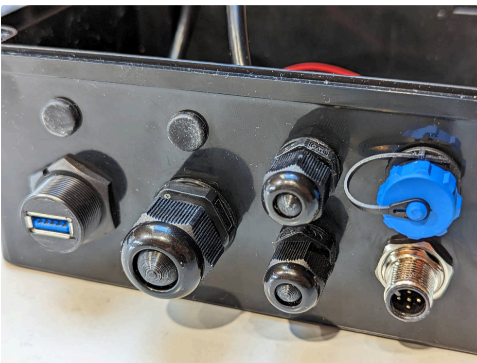
Cable glands installed.
